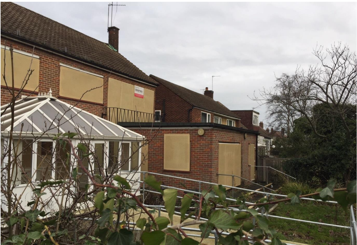
Rear elevation of host building
