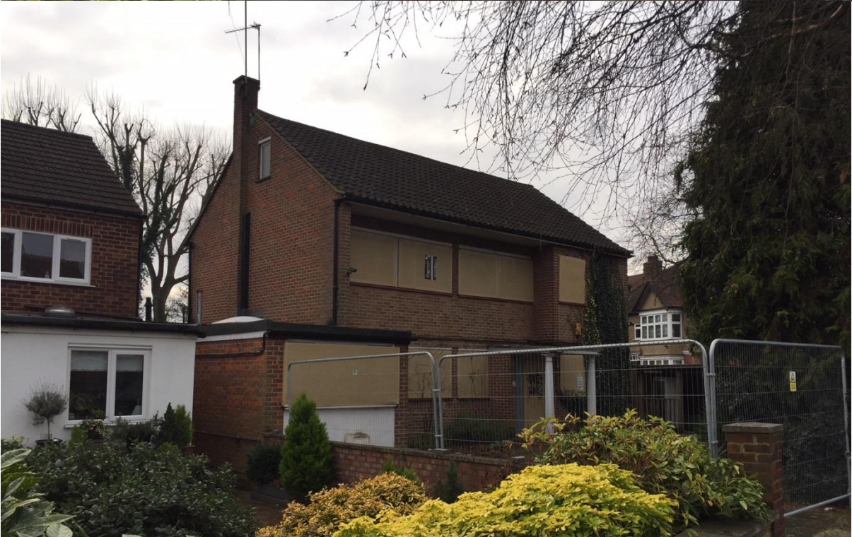
Front elevation of host building, No.44 Flambard Road to the left
