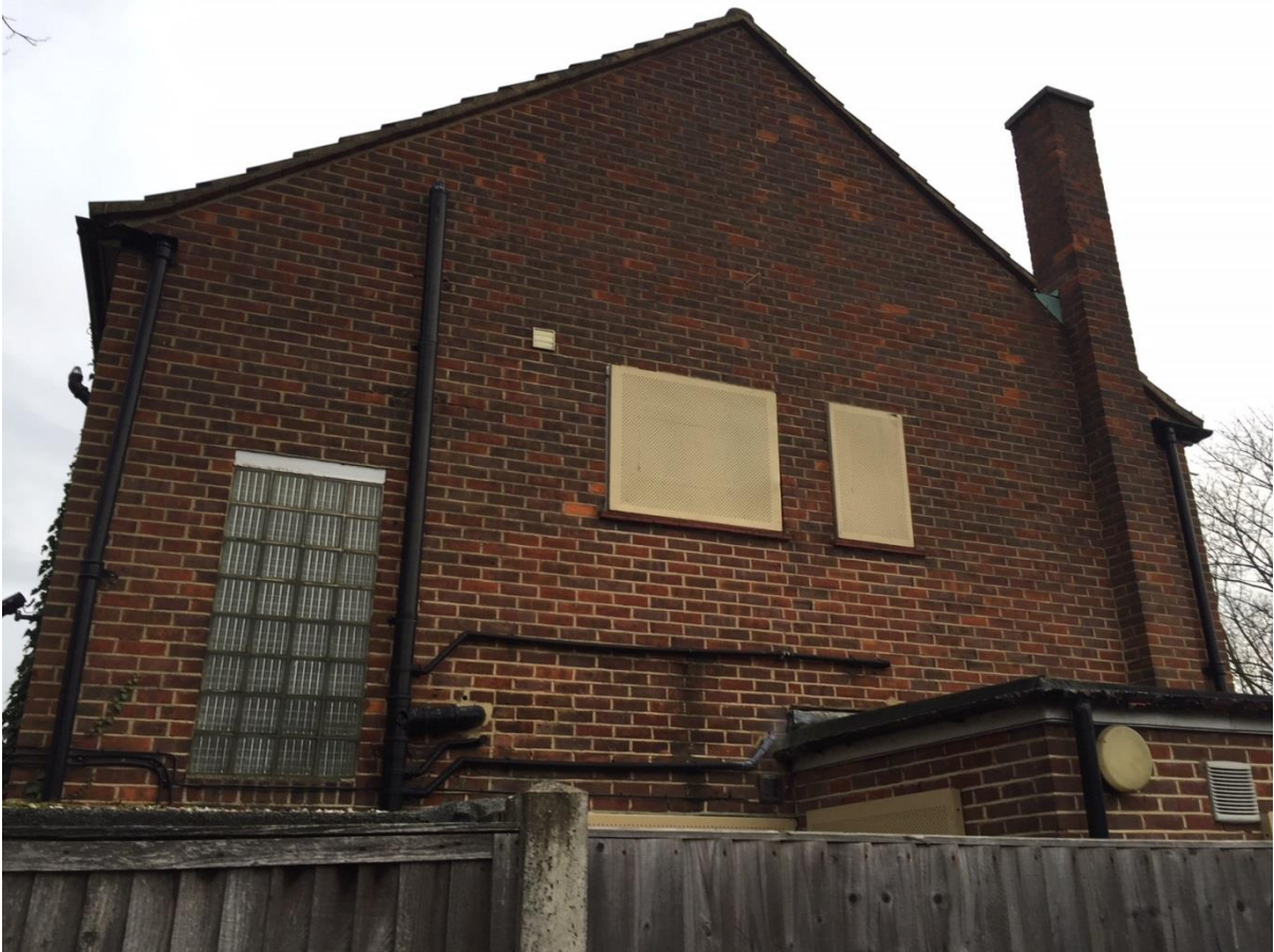
Flank wall of host dwelling
